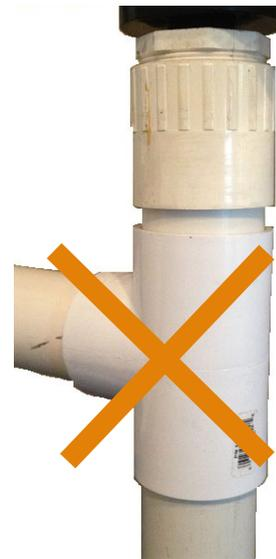
Avoid the use of a tee within the stand pipe. A tee can create false signals that will negatively effect the sensor's performance.
