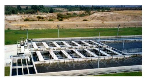
The ClarAtor clarifier equipment is installed into concrete tankage, utilizing common-wall aeration basin construction, helping to lower capital and construction costs.
