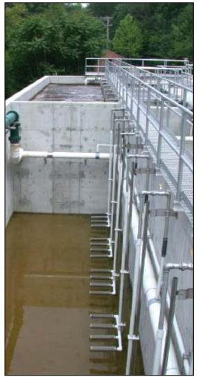
The patented SR (Slide Rail) Diffuser Access System provides simple removal of the aeration diffusers within a tank without turning off the blowers or draining the tank(s). Applications for the system typically are for aeration or digester basins.
