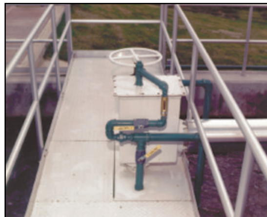
Lakeside's Aeroductor is shown with the air injection line for the eductor tube and air lift headbox on the operator access bridge.
