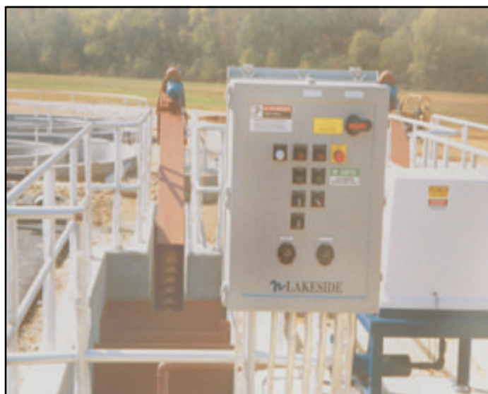
The Inline Grit Collector works well at smaller wastewater plants with peak flows less than 2.0 mgd.
