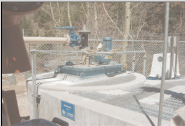
Typical installation of a Lakeside SpiraGrit Vortex Grit Chamber with an air lift system and grit classifier.
