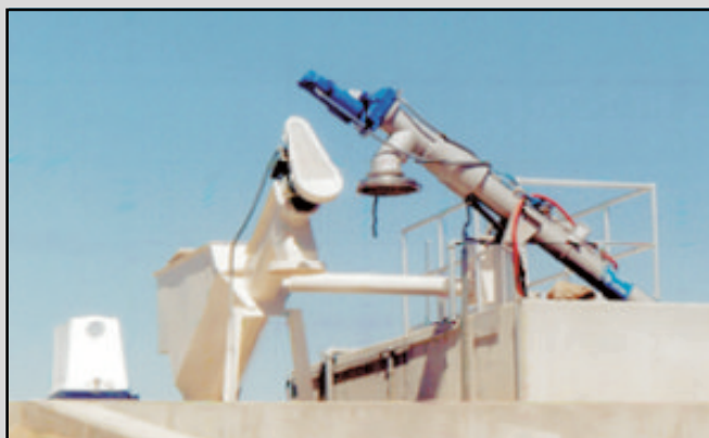
The Lakeside Aeroductor (left) separates grit before directing it to the Model L Grit Classifier (right, shown as part of a plant headworks system).
