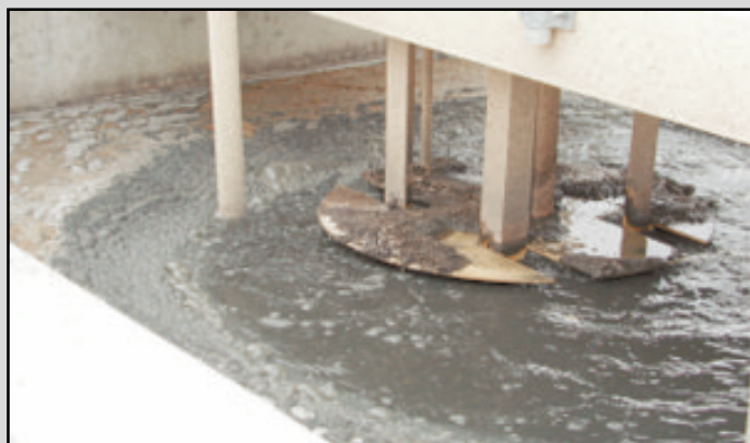
The Lakeside Aeroductor (left) separates grit before directing it to the Model L Grit Classifier (right, shown as part of a plant headworks system).
