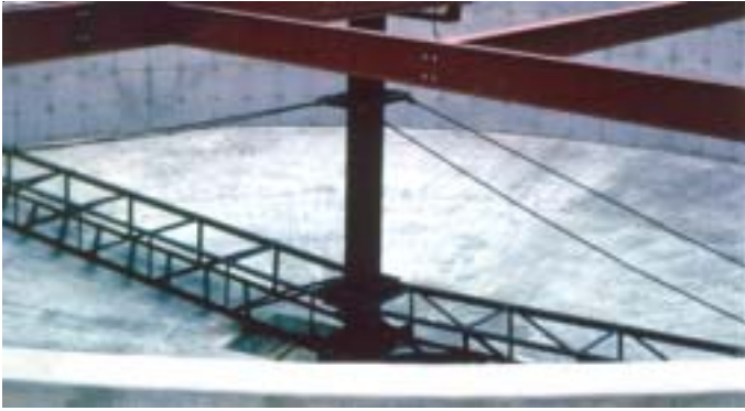
Conventional straight-blade angled scrapers.
